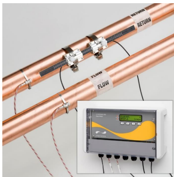
Figure 12 Fully assembled U1000MkII-WM Heat Meter unit
