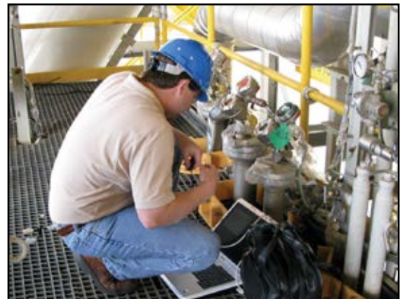
An Orion technician operates PACTware on a drilling rig
