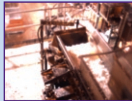
CHUTE PLUG CONTROL
