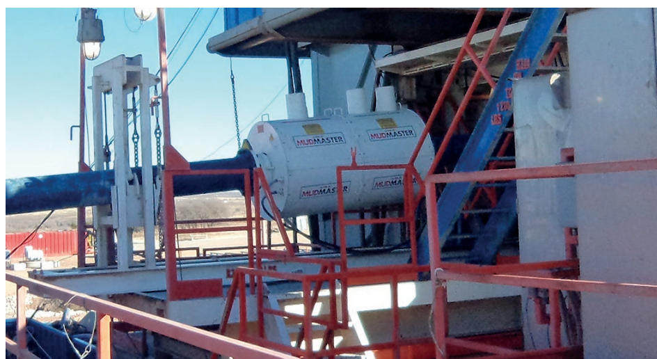
Typical MudMaster™ installation on a 12" gravity fed outlet flow line
