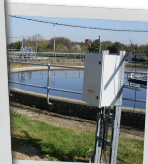
Vertical unistrut mounting near settlement tank
