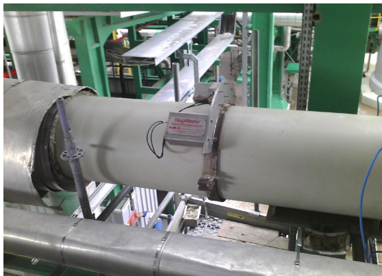
Kashagan Field – SlugMaster Reflexor Transducers
