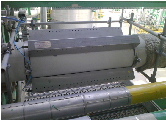
Kashagan Field – SlugMaster Time of Flight Transducers
