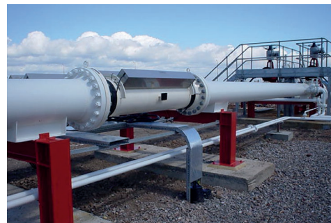
Installed Meter with Protective Shrouds
