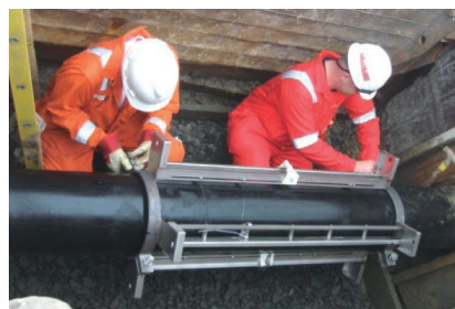
Underground, submersible installation for 56 inch (1425 mm) pipe. Clamp-on sensors are quickly installed, without interrupting flow.
